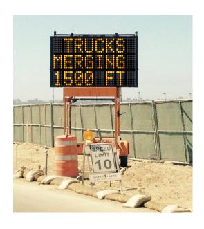
Smart Zone offers remote monitoring and message updating, automatic usernotification via text message or email and is designed to work with any traffic management system.
